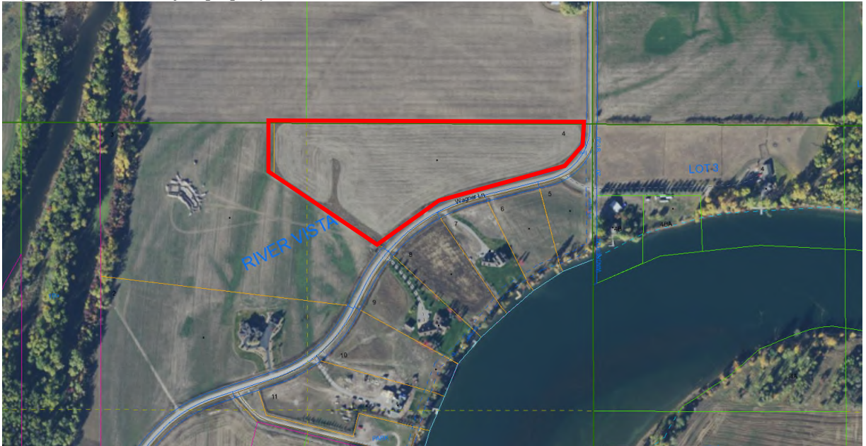
Figure 1: Aerial of subject property outlined in red
