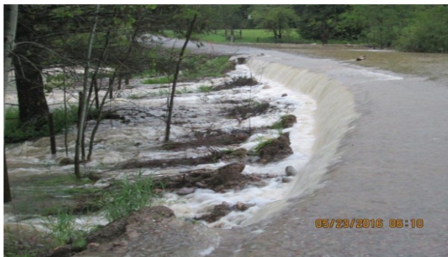
Rabb Road flooding May, 2016
