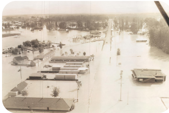
1964 Flooding Strip in Evergreen, MT
