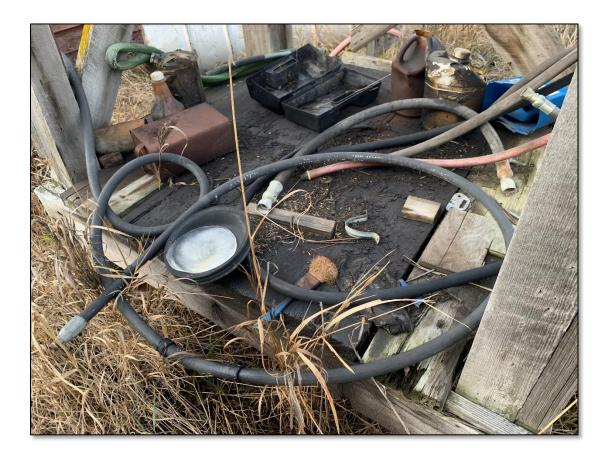
29 | Hydrocarbon-stained platform and waste fluid at the base of an AST stand.
