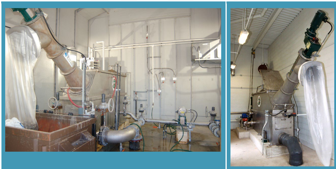
Figure 2. Septage Receiving Example – JWC Honey Monster
