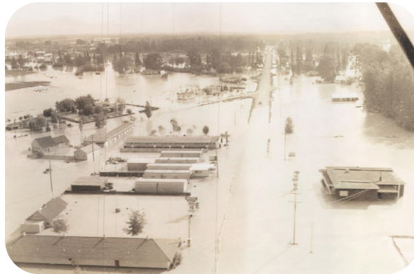
1964 Flooding Strip in Evergreen, MT
