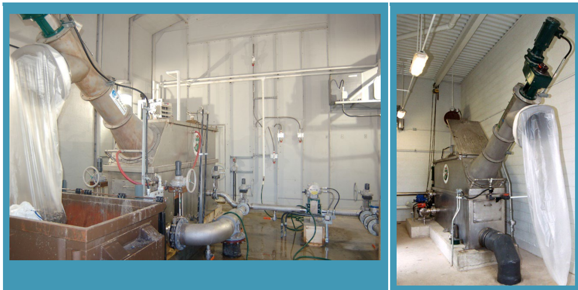
Figure 2. Septage Receiving Example – JWC Honey Monster
