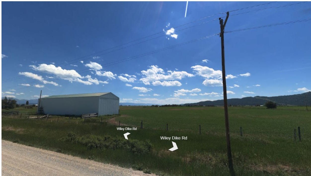
Figure 18. Power Line along Wiley Dike Road. Courtesy Bing Maps
