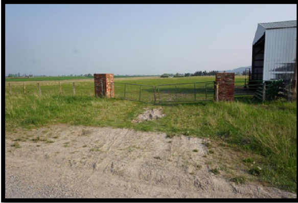
Photo 19 Driveway and Gated Entrance to Subject Property
